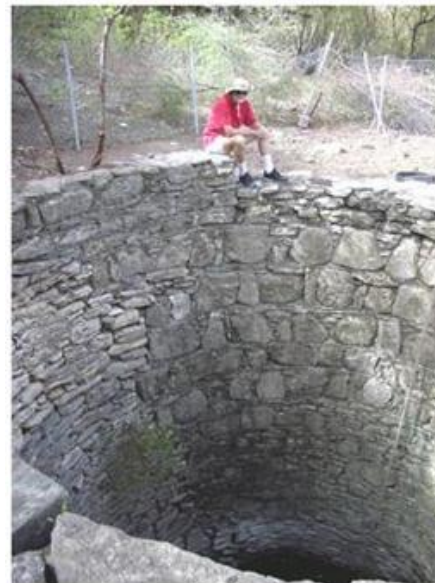
Figure 4.3: The first dug well at Tibeau, Carriacou
