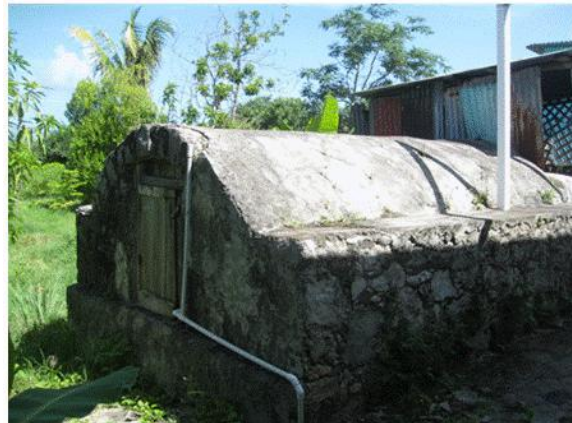
Figure 4.6: Cistern built in the 1870s and currently in use
