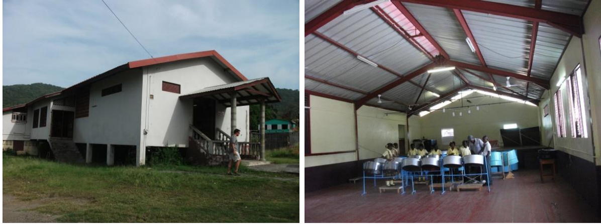
Figure 3.9: Community center / Hurricane shelter
