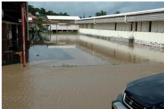
Figure 4.16: Hillsborough Secondary School, Carriacou, flooded during a 2008 event
