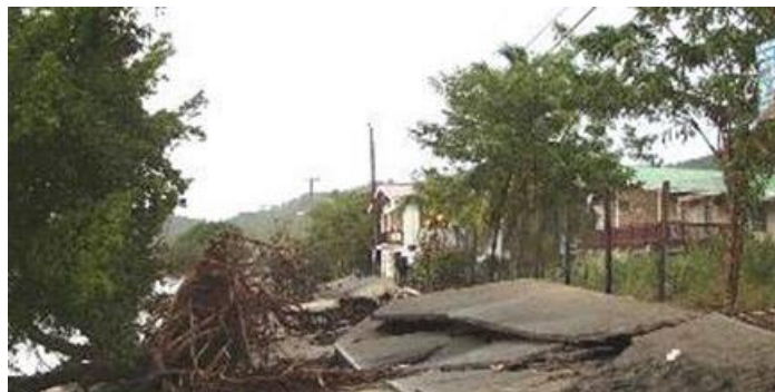
Figure 9.4: Beach erosion at Harvey Vale due to storm surges generated by Hurricane Lenny in 1999 leading to the collapse of a main roadway
